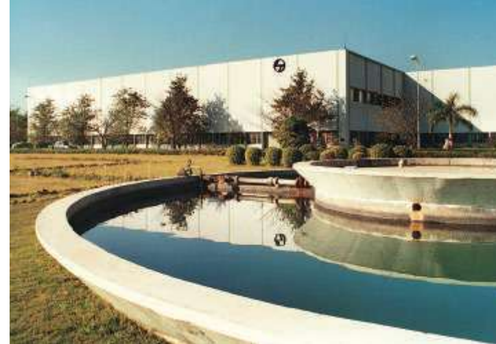
Switchgear Factory, Ahmednagar
