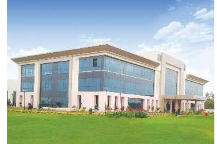
Switchgear Factory, Vadodara
