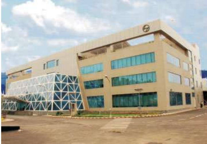
Switchgear Factory, Navi Mumbai
